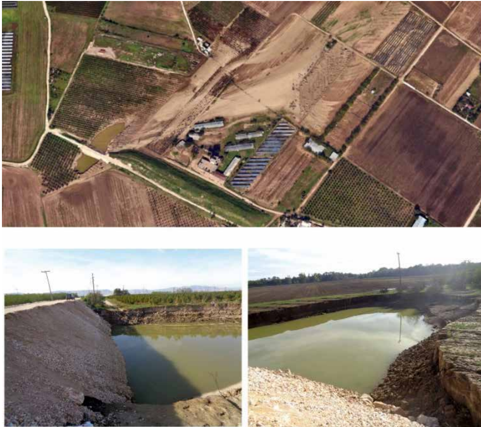
Figure 3. Google Earth scene showing the Kioski failure on October 2023 note on the satellite view the produced basin due to the embankment failure and the deposited material over cultivated lands. The lower left photo shows the restored embankment a few days after the flooding the photograph was taken looking west. The photograph to the right shows the basin at the south of the embankment.
