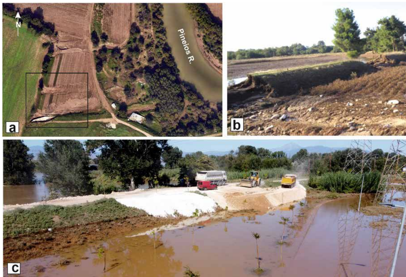
Figure 2. (a) Google Earth scene showing two failed low-height embankments. (b) Field photo of the two failed embankments. (c) The embankment at the DEYAL site was repaired immediately after the flooding. All the localities are at the west entrance of Larissa City, near DEYAL facilities.
