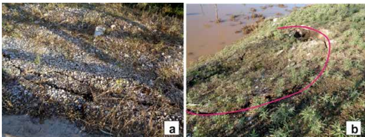
Figure 6 Second order failures of embankments.
