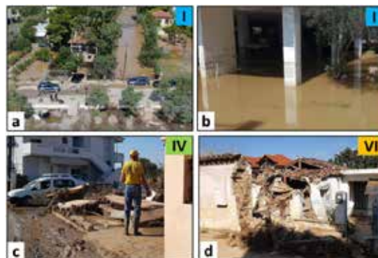
Figure 4. Different flash flood impact severity classes on buildings. (a, b) Garden and pilotis had flooded in Lefkadi beach (Class I). (c) Yard walls and fences suffered from structural damages including total collapse in Vassiliko (Class IV). (d) House suffered from structural damages including failure of supporting elements in Vassiliko (Class VI).
