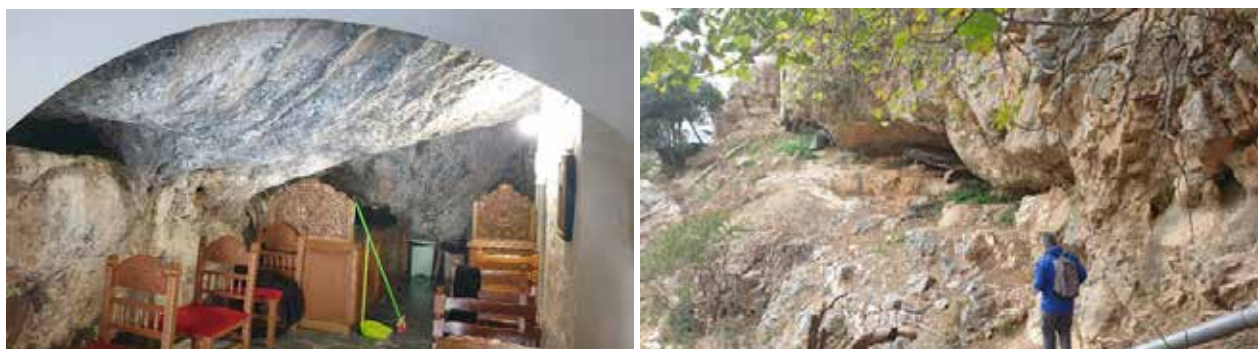
Figure 3. View of the upper low-angle fault surface (No 3, Figure 1 & Figure 2) which forms the roof of the Catholicon (left). View of the lower low-angle fault surface (No 4, Figure 1 & Figure 2), situated at lower elevation than the main foundation level of the Monastery, where minor caves and undermining have formed (right).
