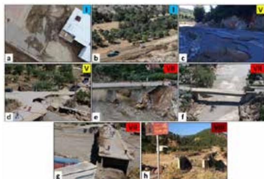
Figure 3. Different flash flood impact severity classes on transportation. (a, b) Inundation of road surface in Vassiliko village (a) and Afrati settlement (b) (Class I). (c, d) Damages to the asphalt surface and levees scoured on the road Afrati - Pissonas (c) and in the Afrati settlement (d) (Class V). (e, f, g) Bridges suffered from structural damages and partial collapses in Vassiliko (e), Filla (f) and Afrati (g) (Class VII). (h) Bridge suffered from complete collapse in the settlement of Mistros (Class VIII).
