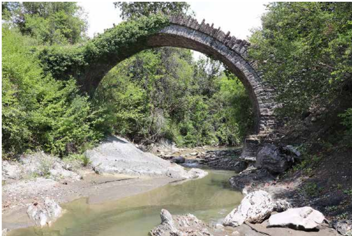
Figure 1. Panoramic view of the bridge. Damage from vegetation and erosion to the foundation can be seen.
