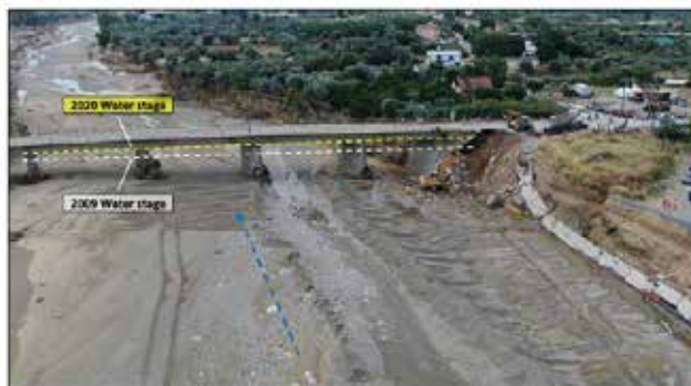
Figure 9. A downstream view of the Vassiliko bridge, illustrating the estimated maximum water levels during the 2009 and 2020 flood events (indicated by white and yellow lines), based on high-water marks identified during post-flood surveys. The blue arrow indicates the river flow direction.
