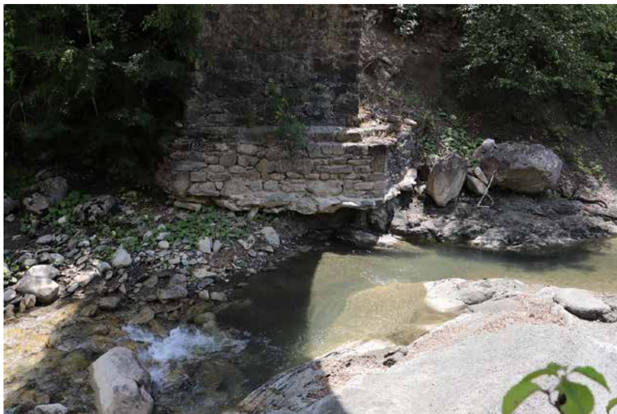
Figure 2. Detail of erosion in the foundation pedestal.
