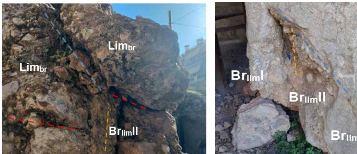
Fig. 5. On the left: Precarious equilibrium conditions in overhanging fractures of the Lim_{br} Limestone and the Br_{limII} Calcareous Breccia on the northern pillar, due to the cross-sectional plane of tectonic discontinuities. On the Right: Detachment of rock fragment from the base of the southern pillar - creation of a local undercrop. The failure occurred at the contact of the Calcareous Breccia II ( Br_{limII} ) and the Calcareous Breccia I ( Br_{limI} ), along discontinuities J2 and J3.
