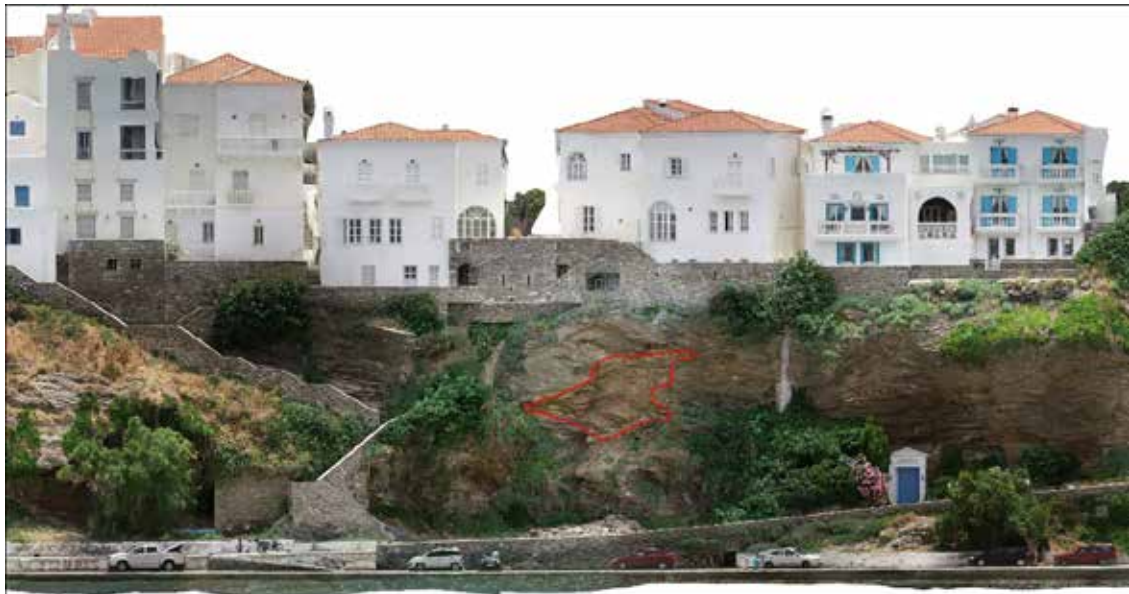
Figure 2. General view of the failed slope, the overlying buildings along the slope crest, and the footpath along the slope toe. The location of the failure is indicated by a red outline.
